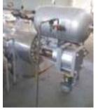
Globe Valve With Pneumatic Actuator for Turbine Protection TGM - CITROSUCO
